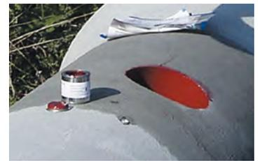
3. Press the pipe connector centrically – with its mark in axial direction of the pipe – into the bored hole until the stop is reached. Central insertion is important, in order to compress the first rubber rib evenly and to avoid its turn over.
