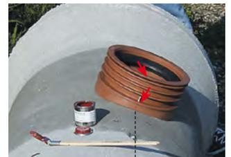
4. Before the mounting of the connection pipe **DS BAST GV** has to be applied on the sealing ring in the socket of the connector and on the pipe spigot end. In case of a cut pipe its end has to be bevelled before.
